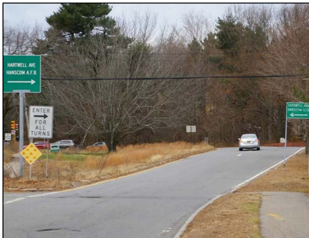
Conflicting wayfinding signage at jug handle entrance.
