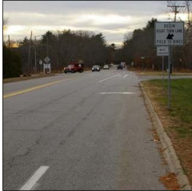
Confusing lane markings along Hartwell Avenue southbound.
