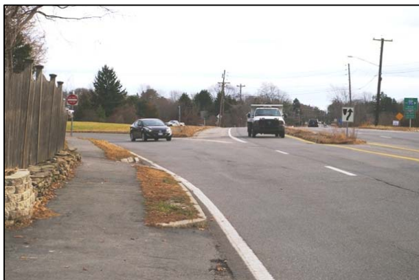
The I-95 southbound off-ramp merging with Bedford Street westbound.
