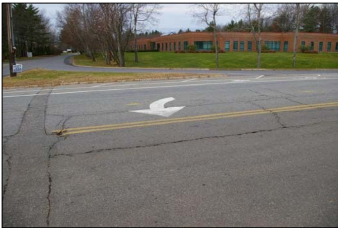
Incorrectly marked left turn lane.
