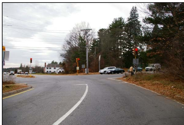
No lane designation signage or markings at the jug-handle southbound approach.
