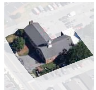
CENTRAL FIRE STATION
