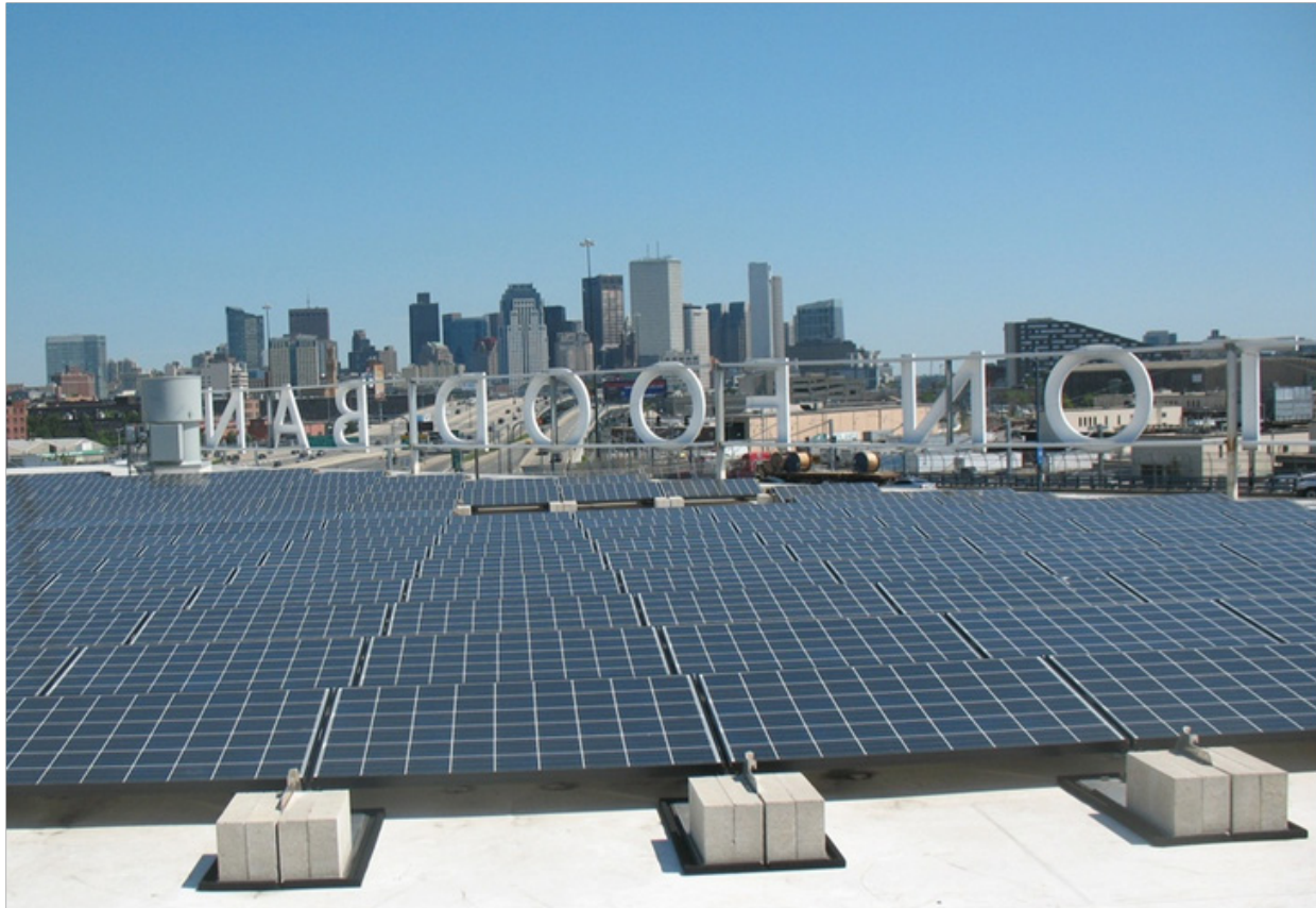
Image: The Greater Boston Food Bank’s solar panels, available at Massachusetts Energy & Environmental Affairs photostream, http://www.flickr.com/photos/masseea/5857332148/
