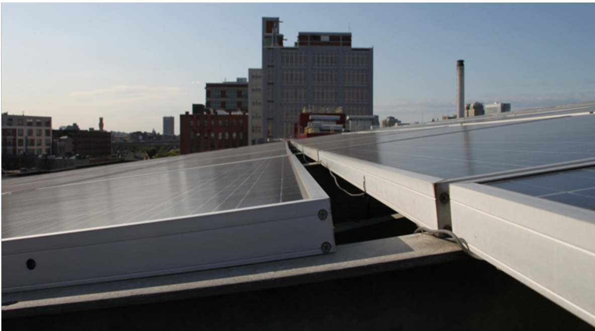
Image: This 49-kilowatt photovoltaic system atop the Artists for Humanity EpiCenter in Boston generates 50% of the building's electricity needs, available at Massachusetts Energy & Environmental Affairs photostream, http://www.flickr.com/photos/masseea/6260744813/
