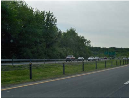
3 Cable CASS System on Route 213
