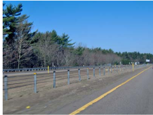
4 – Rope Brifen System on I-495
