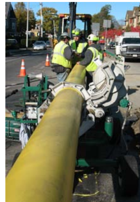
Plastic pipe being installed on a street outside Boston.
