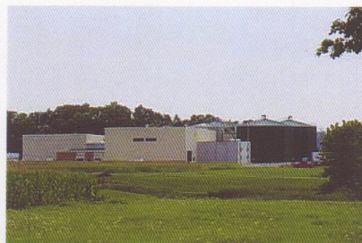
Fremont, Michigan USA Food Waste Facility (Courtesy Biomass Magazine)
