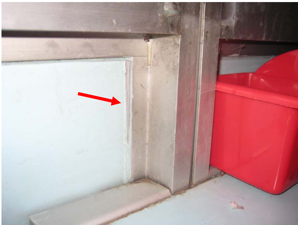
Figure 1 Primary Source Caulking on Interior Panel within Window Frame
