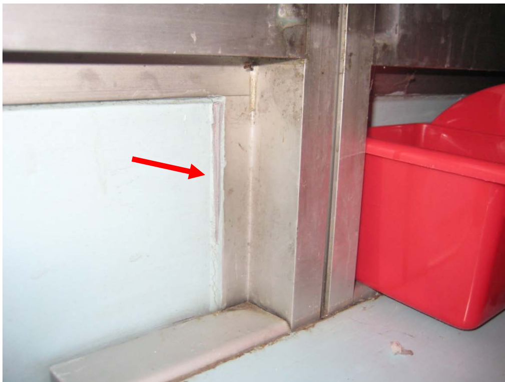
Figure 1a Primary Source Caulking on Interior Panel within Window Frame
